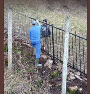
Phase 3: Construction of gate continued
