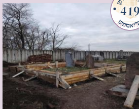
Picture of the new foundation poured on the original foundations
