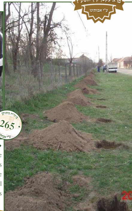
→ Preparing the foundations for the fence at the original borders
