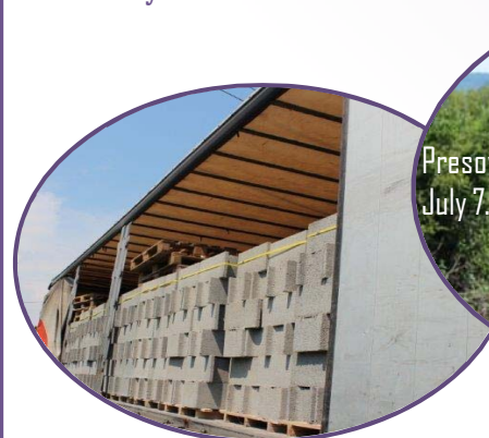
Transport of material for the final phase of fence
