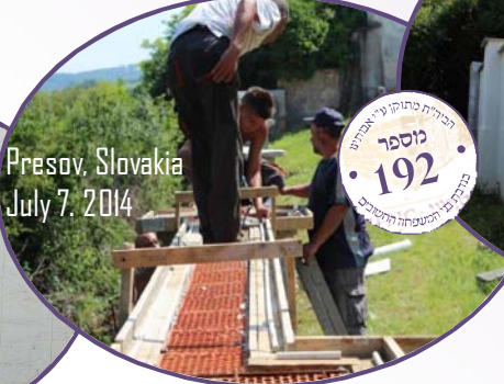
Construction of the impressive fence
