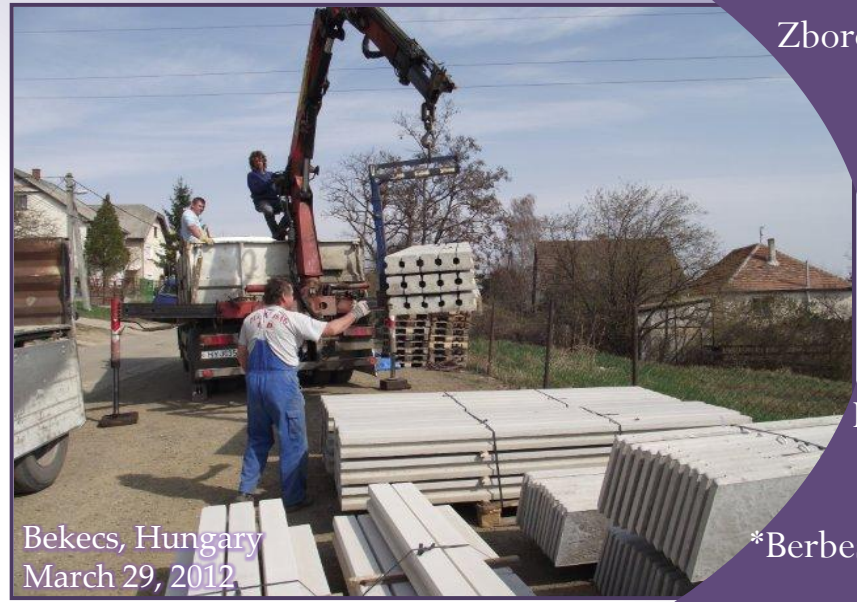
Material for fence arrives to site; foundations for fence are erected
