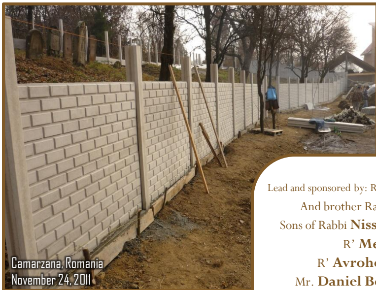
Front section of fence completed
