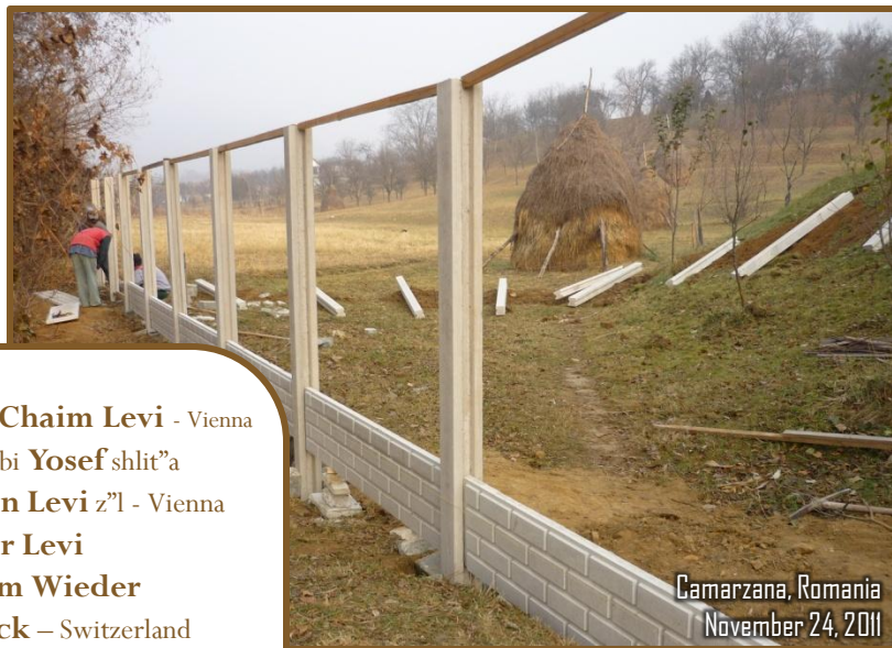
Digging the foundations for the fence
