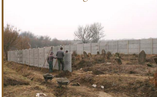
Constructing the fence
