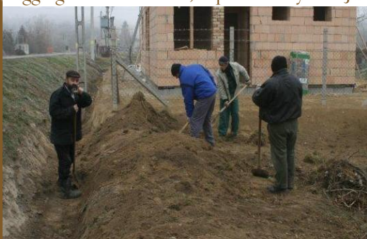
Digging the fundaments, supervised by HFPJC
