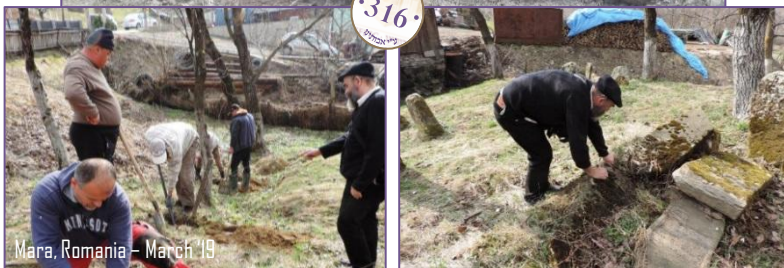
Foundation for fence being set up
