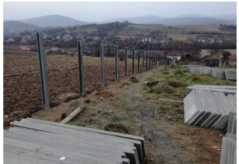
Foundations for fence being laid
